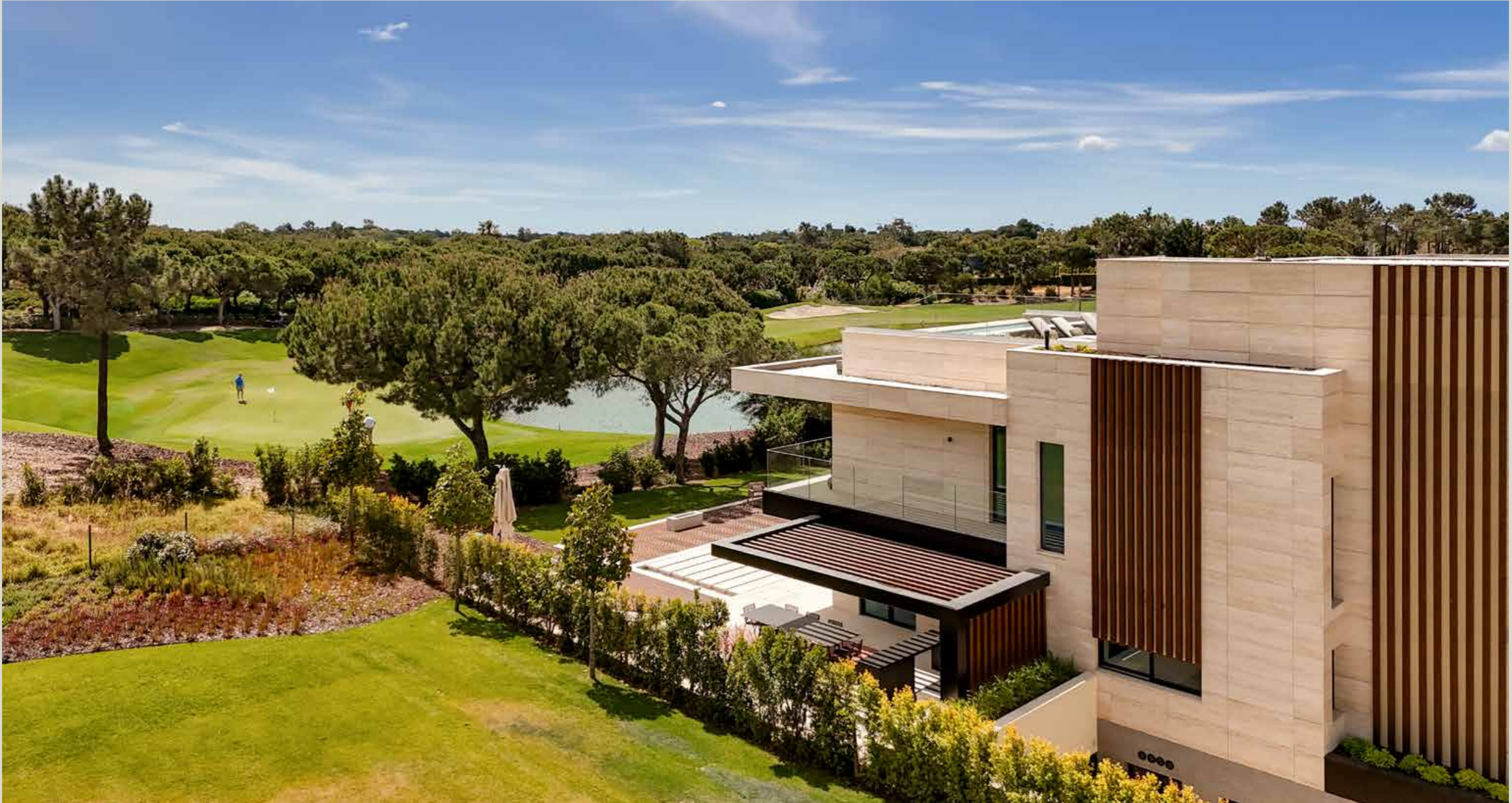
Above; Horizon Residence - Show Unit
