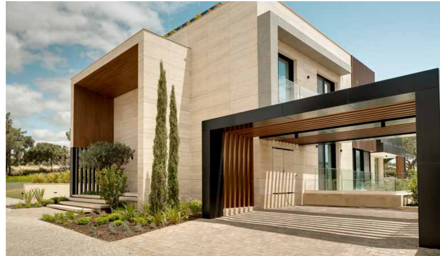
Above; Horizon Residence Show Unit
